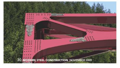
The design team used built-up box members and HSS sections to create a neat and clean appearance. These built-up members, with top and bottom chords, are connected with minimally-obstructive, slender hollow structural section tube web members.
